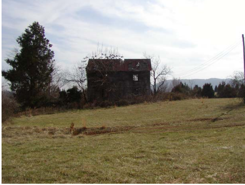
Circa 1870 – 1890 framed house located on edge of Kirtley facing north
